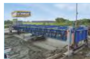
Concrete Road Paver
