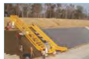
Concrete Canal Paver
